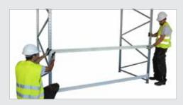
Position a pair of frames. Hold them in place with a pair of beams.
